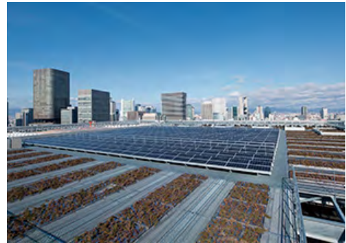
On the roof of the east building of the Nippon Life Head Office
