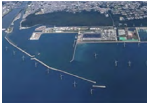
Offshore wind power station (source: Akita Offshore Wind Corporation)
