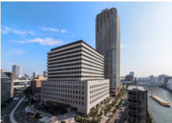
Exterior of Nippon Life Hospital
