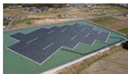
(Solar power plant operated by Kyocera TCL Solar LLC.)
