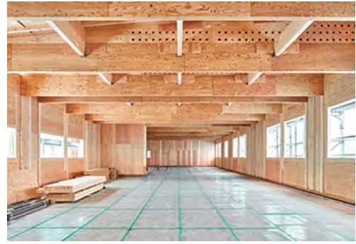
Chiryu Sales Office
