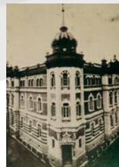
Former corporate headquarters (1902-1959)
