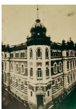
Former corporate headquarters (1902-1959)
