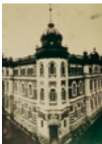
Former corporate headquarters (1902-1959)
