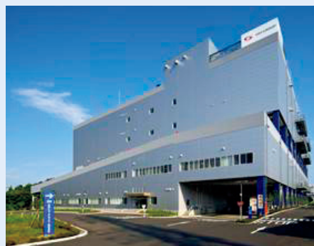
Exterior view of Atsugi Logistics Center
