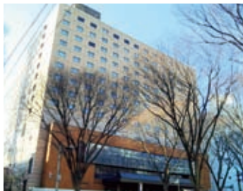
Exterior of the former Sendai Excel Hotel Tokyu
