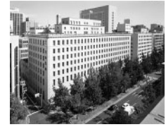
Current head office building
